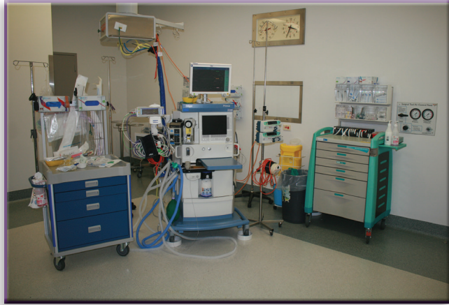
FIGURE 3 Draeger anesthetic machine fitted with sevoflurane and desflurane plenum vaporizers at the Wollongong Hospital in Australia.
